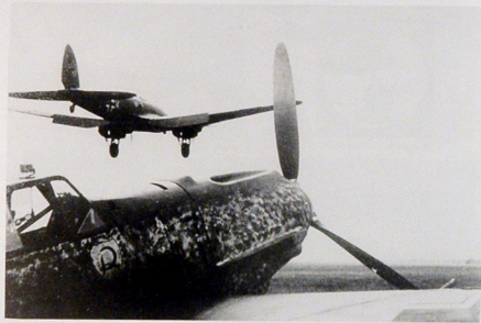
LEFT AND BELOW: Two photographs showing a visiting He 111 landing at JG 2's airfield at Otterville in early August 1940. Of note on the JG 2 Bf 109 in the foreground, is the heavily applied 'stipple' mottling over the RLM 65 on the fuselage side and the motor car type rear view mirror mounted on the canopy framework.
