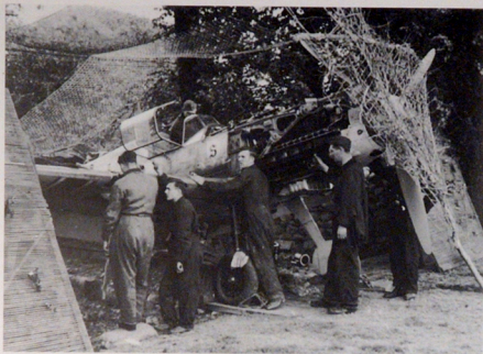
RIGHT AND BELOW: BE 109s of 6./JG 26 receive attention from the ground crews at their dispersal at Marquise - where they arrived from Germany on 21 July 1940. Note the camouflage netting and the tarpaulins tied over the lighter coloured paint on the aircraft noses which have probably been used as a measure of concealment.
