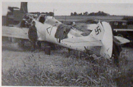
ABOVE AND ABOVE RIGHT: In these two photographs, Oblt Werner Bartels' Bf 109 E-1 has now been raised and had its undercarriage extended in preparation for removal from the site of its forced landing.
